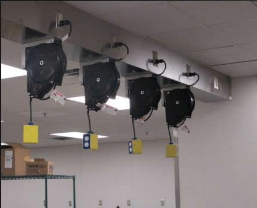
THE KITCHEN LEASH IS DESIGNED SPECIFICALLY FOR AREAS MOISTURE SENSITIVE AND WHERE POWER CORDS NEED TO BE KEPT OFF THE FLOOR PROVIDING WATER-TIGHT ELECTRICAL POWER FOR KITCHENS AND FOOD PREP AREAS.
